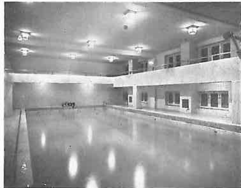
Fig. 3. X-Ray reflectors and Mazda lamps lighting a Swimming Bath. The reflectors are equipped with the second of the two lanterns shown in Fig. 2.
