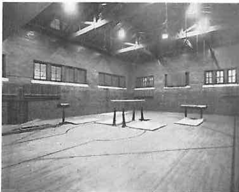
Fig. 1. Gymnasium lighted with X-Ray reflectors and Mazda lamps fixed close to the ceiling.
