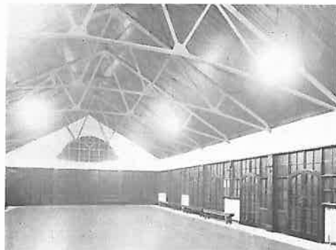
Fig. 4. Mazda lamps and B.T.H. reflectors in large Recreation Room. Note the uniformity of the illumination.
